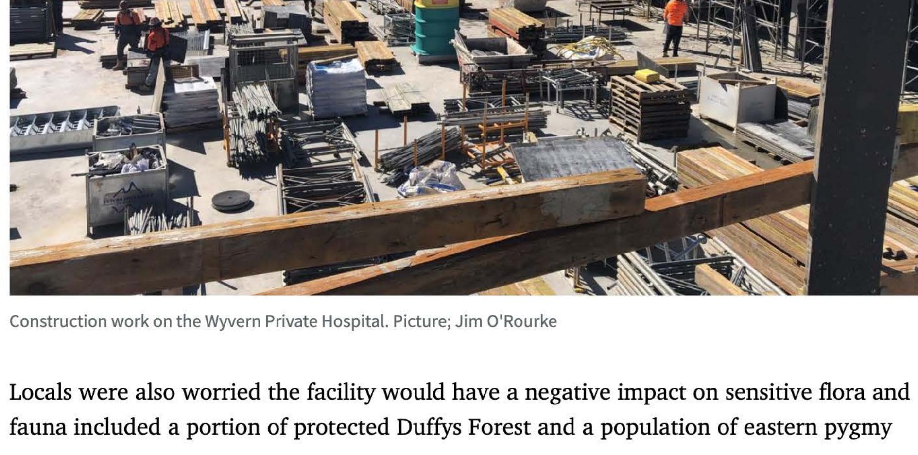
Construction work on the Wyvern Private Hospital. Picture: Jim O'Rourke
