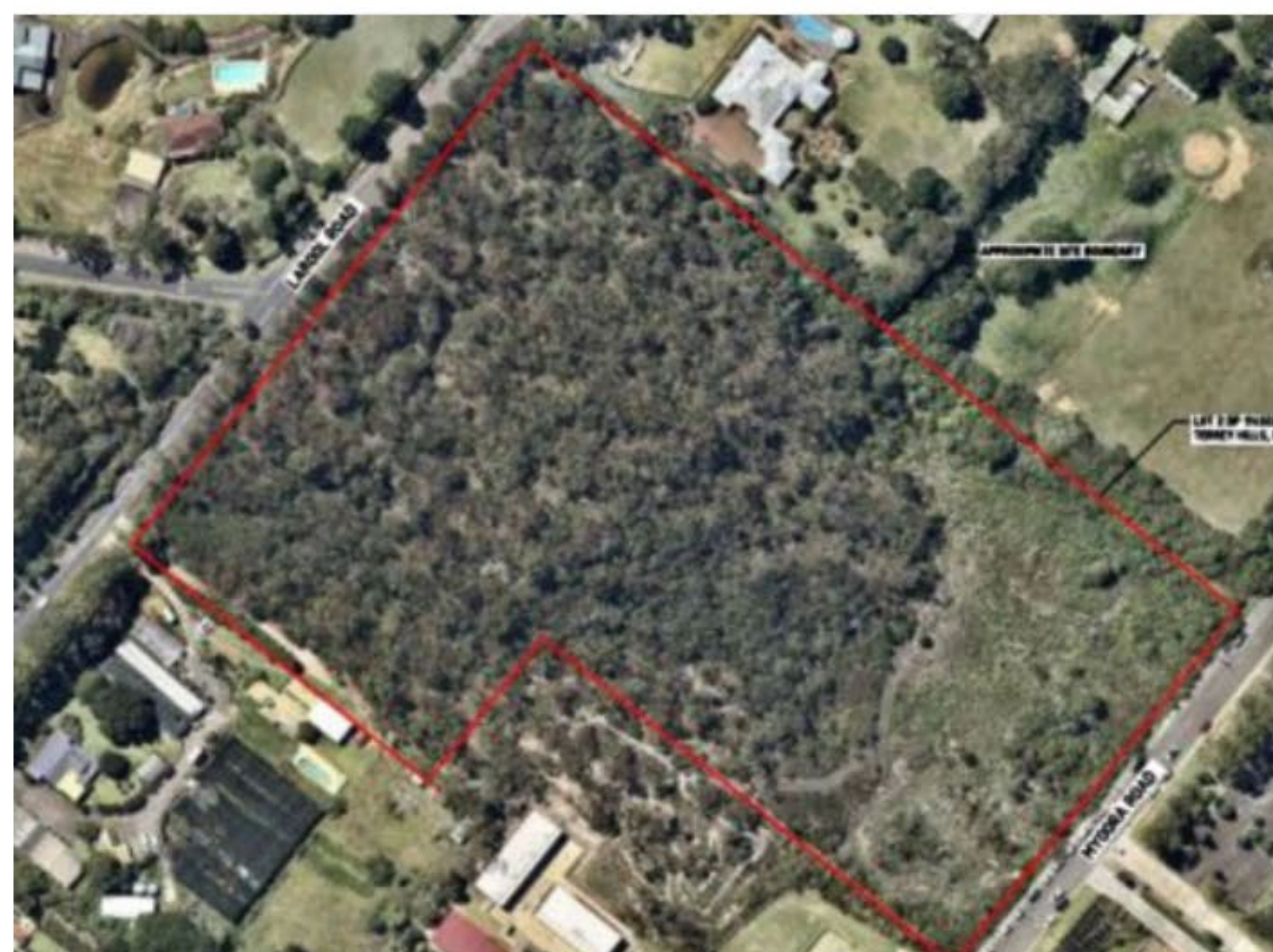
The boundary of the Wyvern Private Hospital site, between Myoora and Larool roads at Terrey Hills. Picture: Martens & Associates
