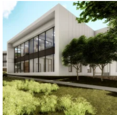
Wyvern Private Hospital, Terrey Hills, is due for completion in mid-2023.
